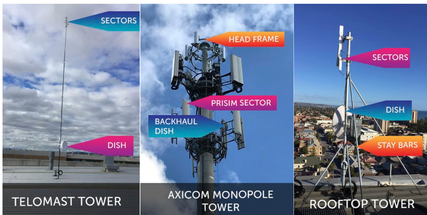
Figure 3.6 Uniti Wireless Tower Solutions
